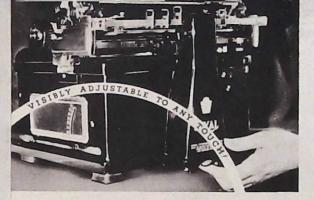
TOUCH CONTROL ... exclusive feature of the new Royal. Operates as simply and easily as a station is dialed on your radio. The key action of the new Royal is instantly visibly adjustable to any degree of touch. Complete adaptability of the machine to the individual touch of the operator, assuring the maximum of comfort throughout the working day.
